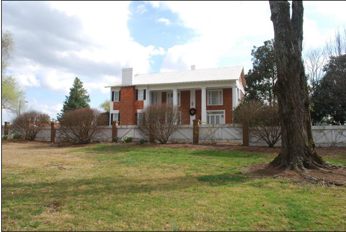
Magnolia Place from edge of pavement of Exit 103 on-ramp.
